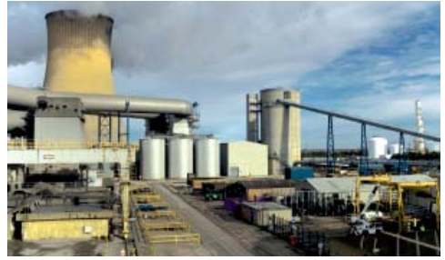
British Energy, Eggborough Power Station, North Yorkshire, UK
