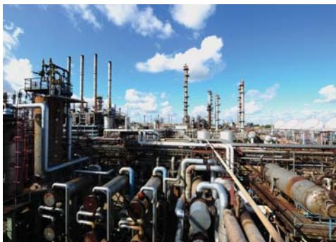
Fawley refinery, Southampton, UK
