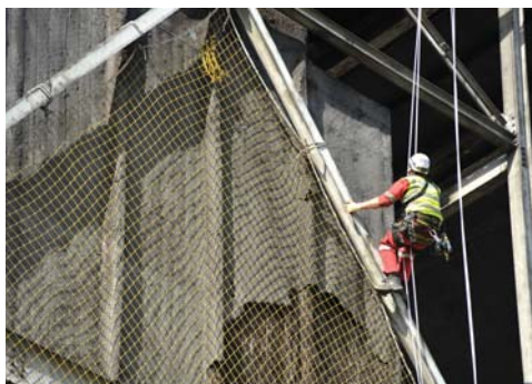
Rope access services, Longannet power station, UK
